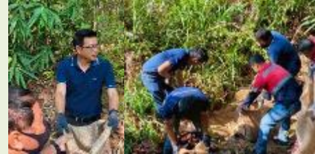
The SCSC Volunteer Project by building a check dam to promote environmental sustainability.
